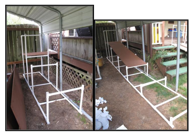
Above, **building framework** of actual ramp section by section. I propped up the plywood on top of various things to figure out heights of PVC "upright legs" at various intervals. Right photo shows first plywood ramp section put on, I later added another upright leg at the end of it to support the top of the plywood section not yet put on. I didn't glue any of the bottom support together until the whole bottom was finished and correctly fitting.
