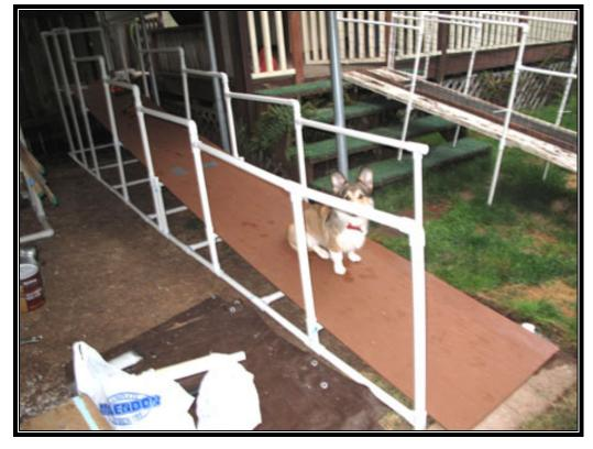
Right, fencing ziptied on to framework. Zips will eventually degrade from UV damage so occasionally have to be checked and replaced.
