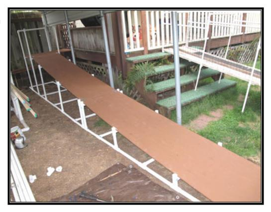
Right, most of PVC framework for sides now installed. For now I'm not going to glue them. The end of the ramp rests on blocks, not on the ground, to help prevent rotting (it rains here a lot).
